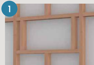
1 Rough-In timber framing to support niche - Ref (Niche Rough-In Guide)
