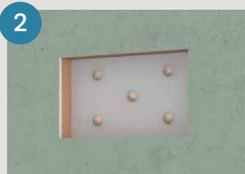
2 Fix Gib / Villa Board, dry fit niche, remove and apply adhesive
