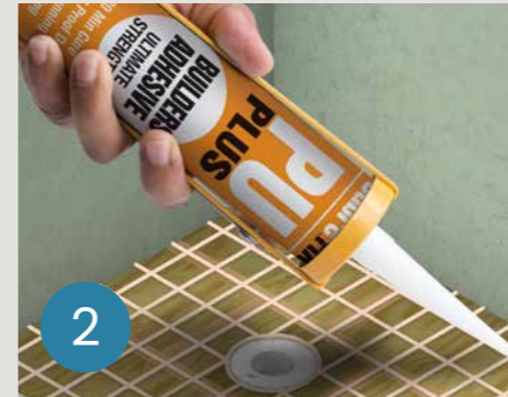
APPLYING POLYURETHANE ADHESIVE
